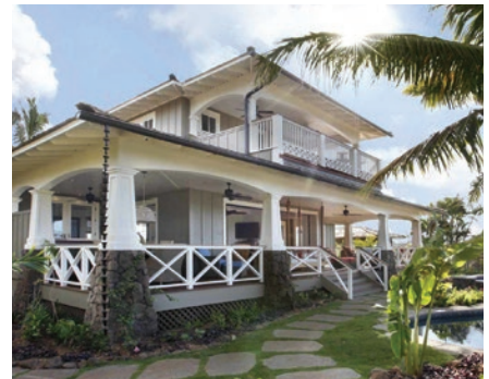
New Home Construction: Kukui'ula - Kaua'i Project
